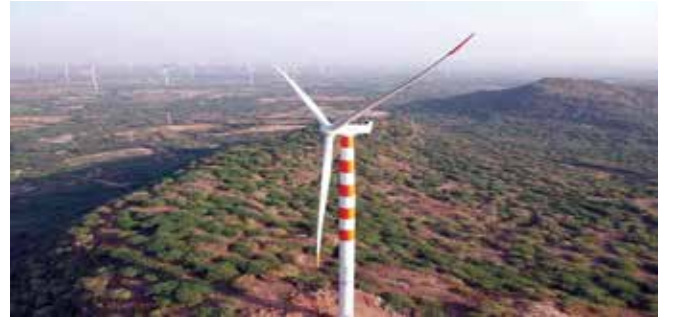
50 MW Wind - Erection of Windmill at Gujarat
