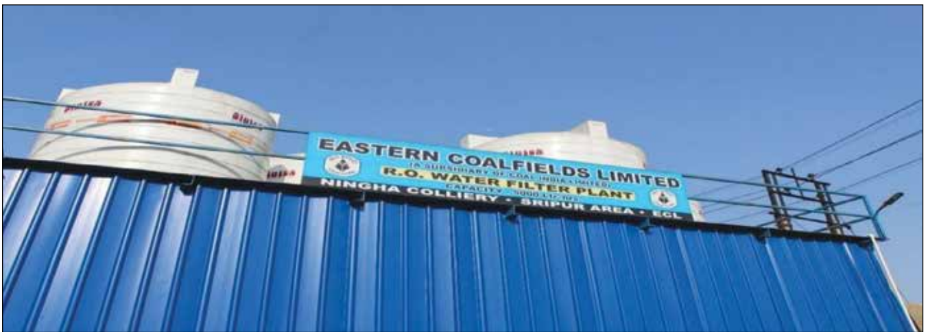
Mine water treatment facility at ECL
