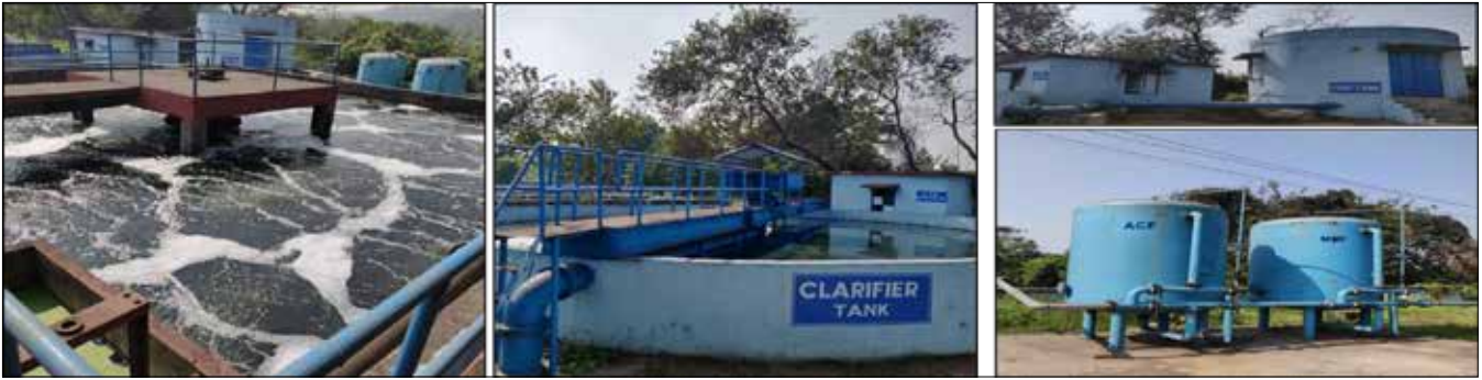
Fig. Sewage Treatment Plant (1.7 MLD), Lakhapur OC, MCL
