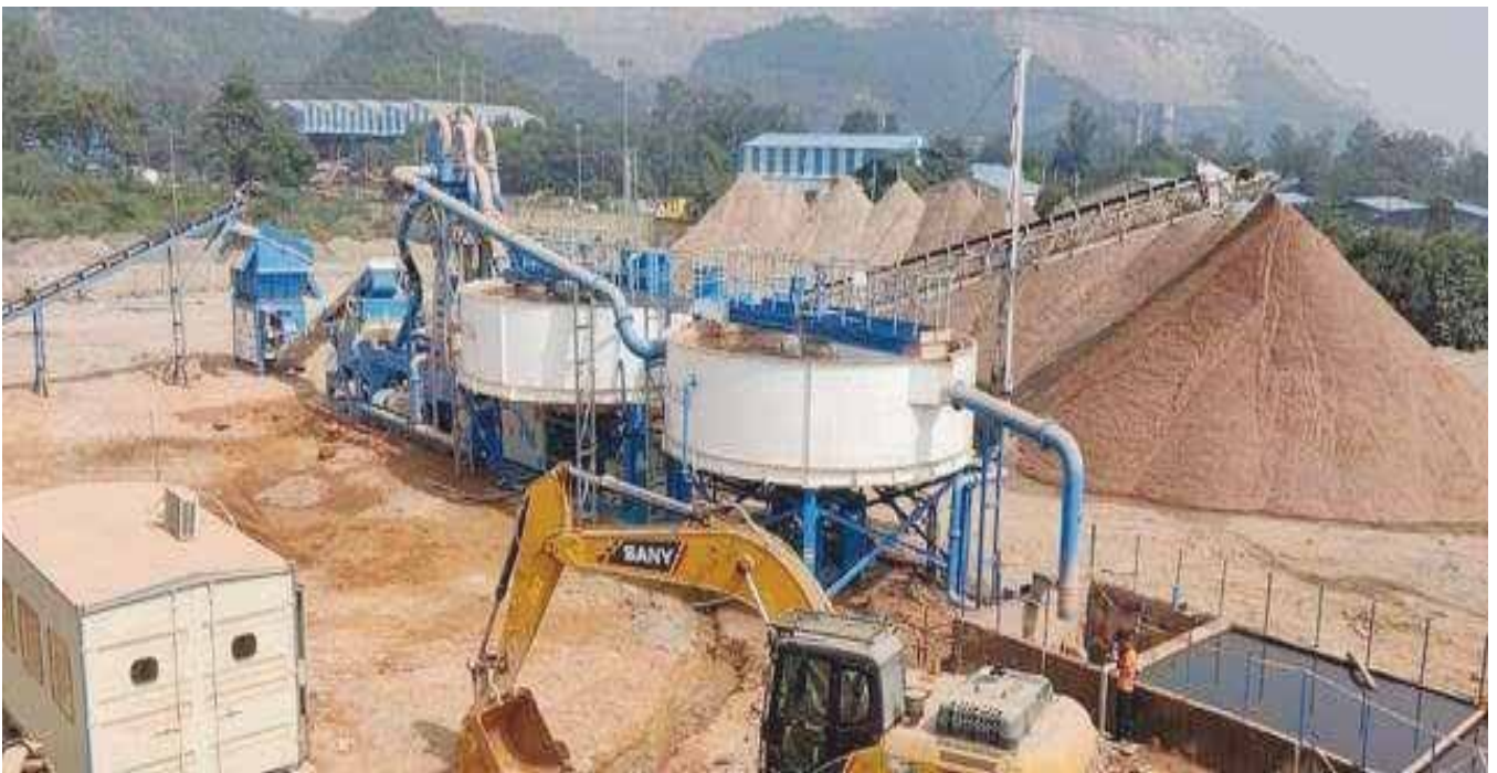
OB to Sand Plant at Amlohri, NCL
