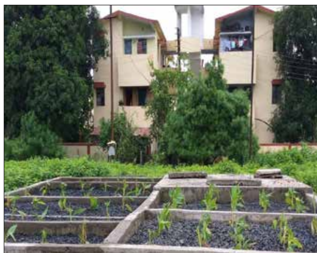
Fig. STP with Phytorid Technology at Umrer Township WCL
