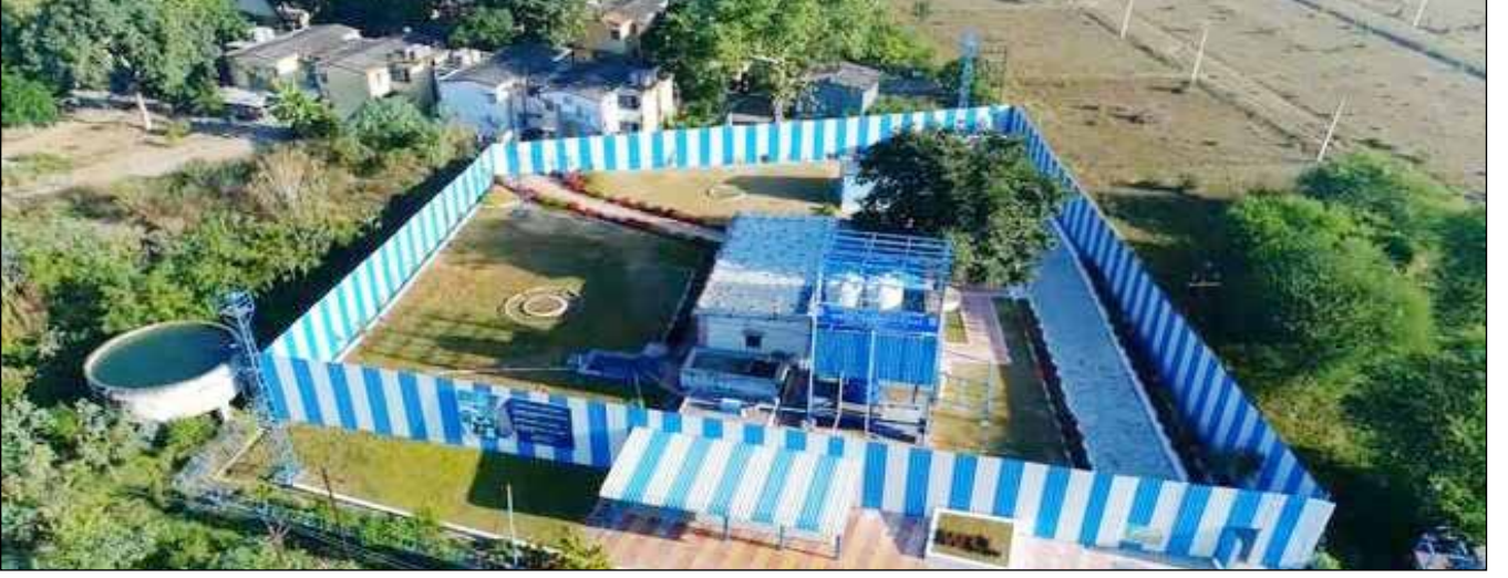
R.O. Plant Facility at WCL
