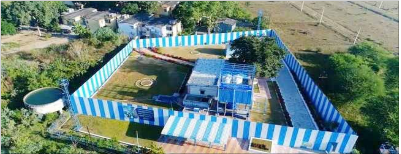
R.O. Plant Facility at WCL
