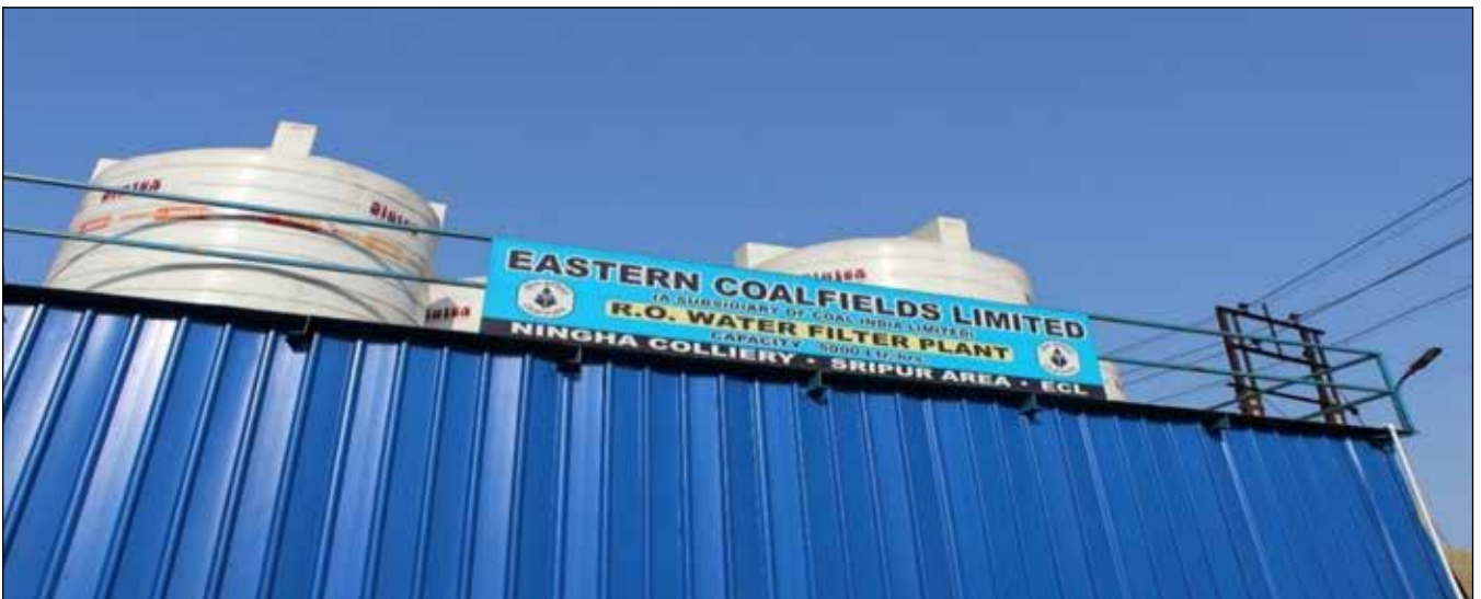
Mine water treatment facility at ECL
