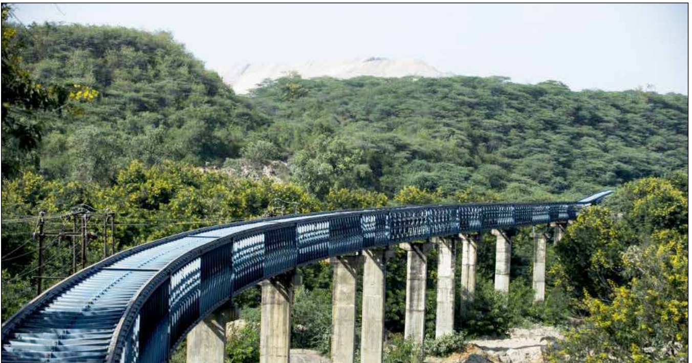
Fig. Krishnashila OC of NCL: Belt Pipe Conveyor
