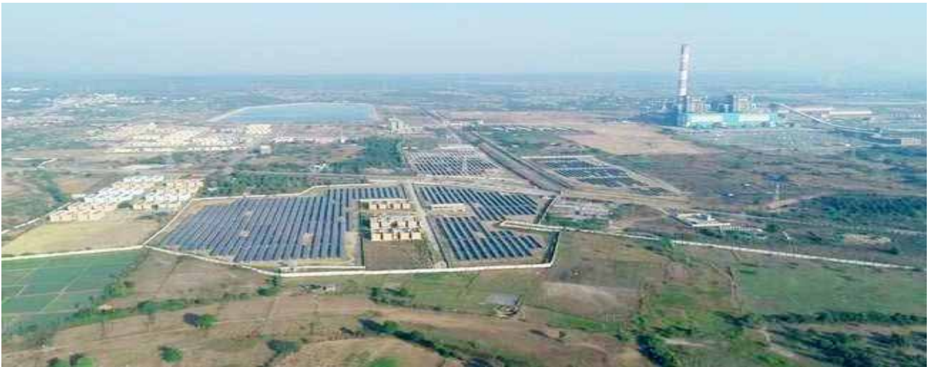
Fig. Solar Power Plant at STTP (10MW)
