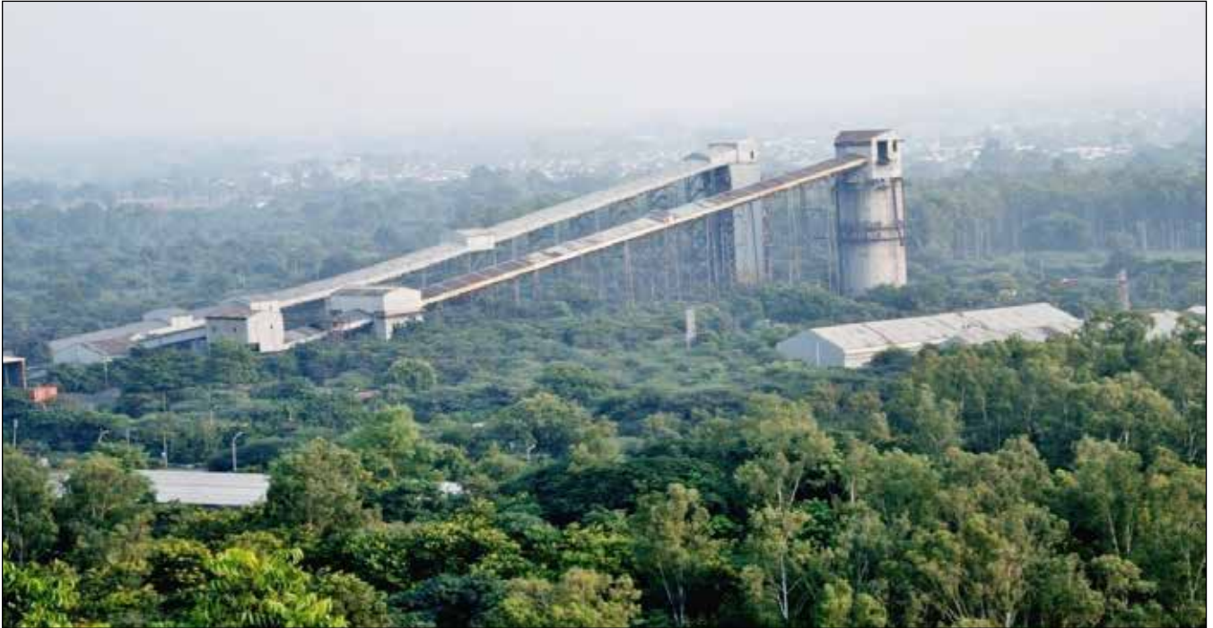
Fig. Nigahi OC of NCL: Closed Belt Conveyor System and then rapid loading system
