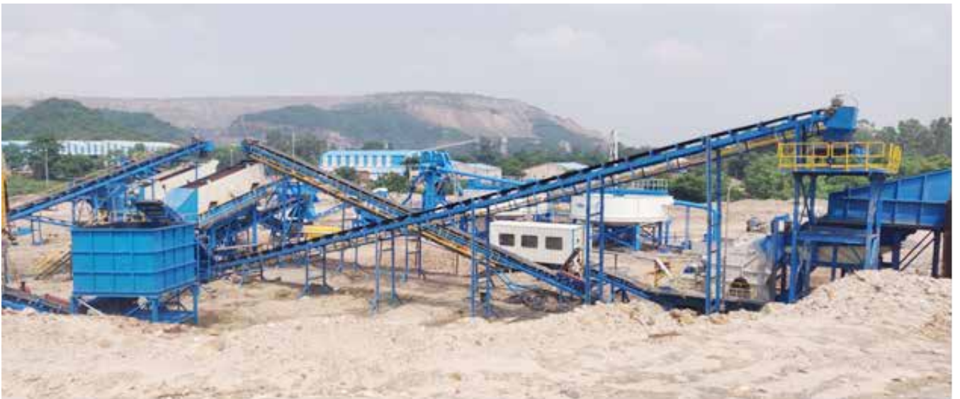
Overburden to M-Sand Plant at Amlohri Plant, NCL
