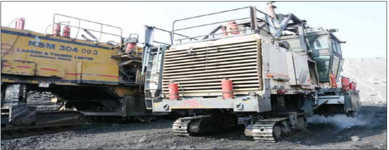
Fig. Surface Miner with water jets, Gevra OCP, SECL
