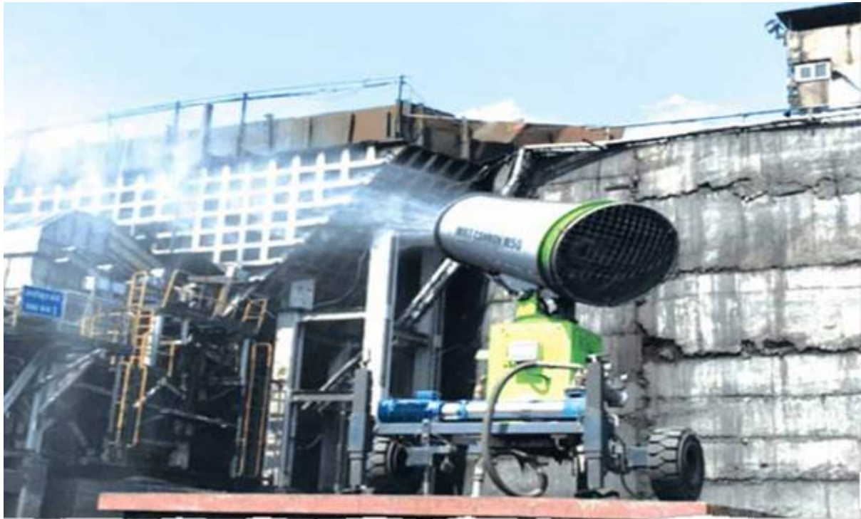
Fig. Mist Gun operation to control dust
