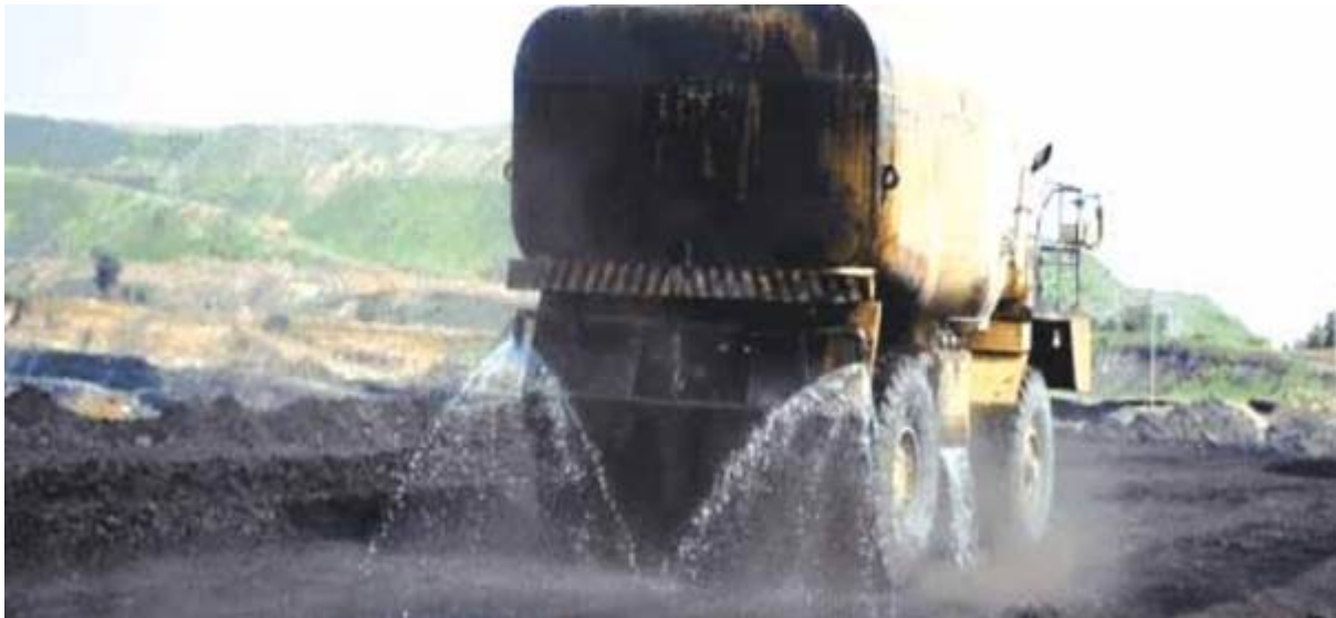
Fig. Mobile sprinklers in operation for suppression of dust
