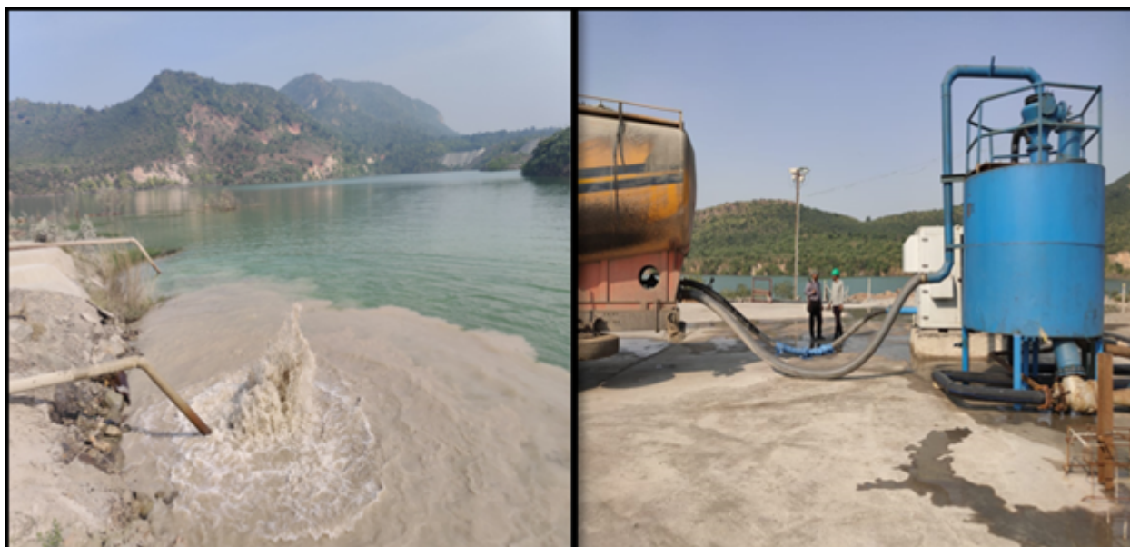
Fly Ash filling in Gorbi Mine (Pit-1), NCL
