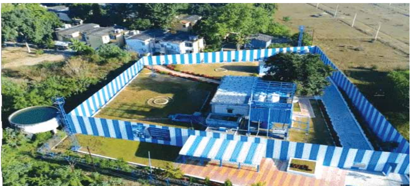
Fig. RO Plant Facility at WCL
