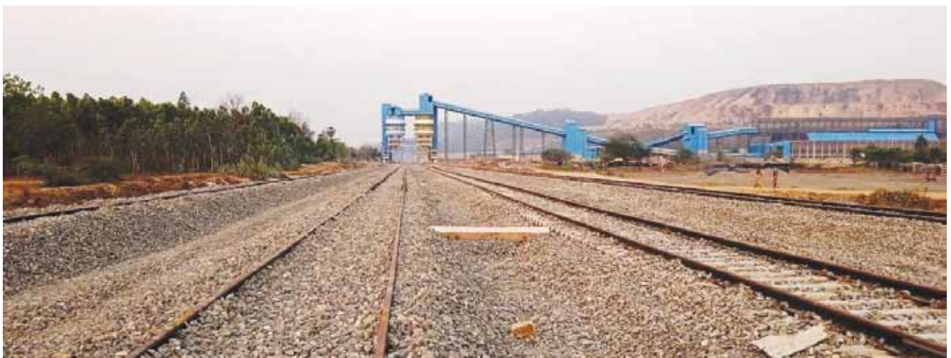
JVR OC CHP and railway line- Development of Infrastructure for Coal evacuation:
