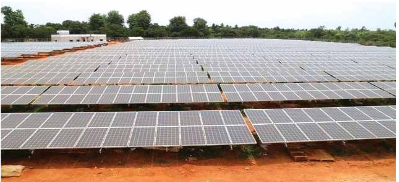
Fig. The flat panel Multi / Poly crystalline silicon PV cell technology in Neyveli Township Block-4
