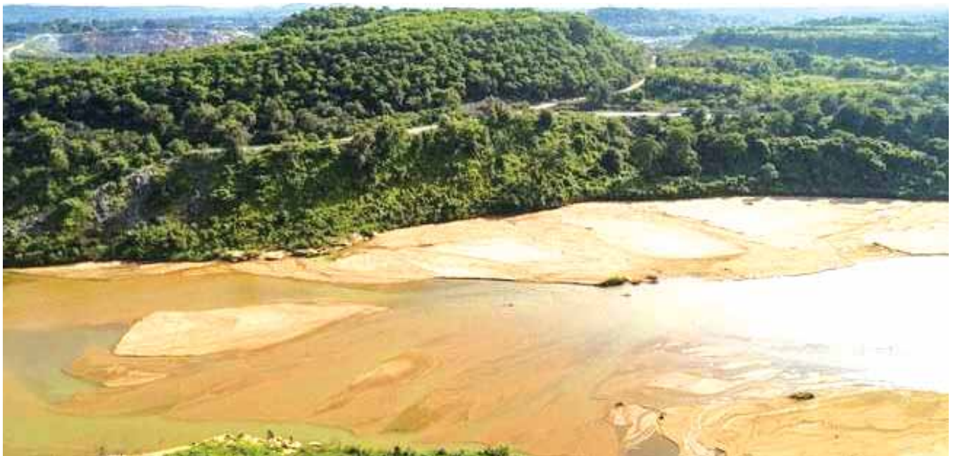
Fig. Green cover developed by CCL along embankment of Damodar River in NK Area
