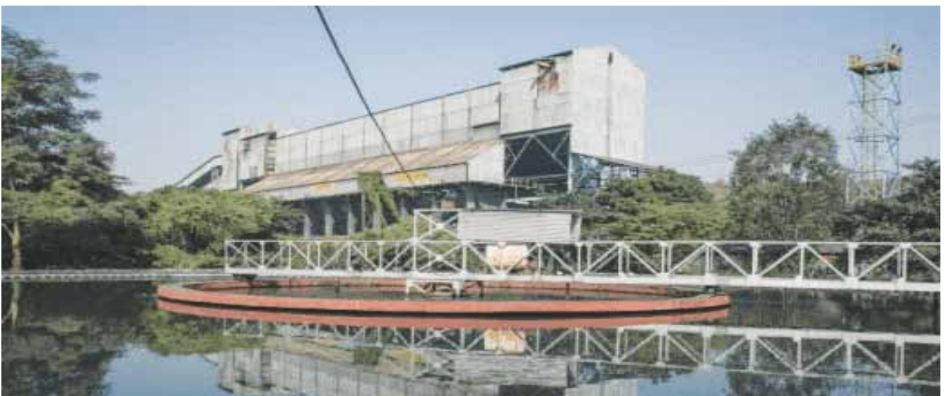
Fig. ETP at Kakri OCP, NCL
