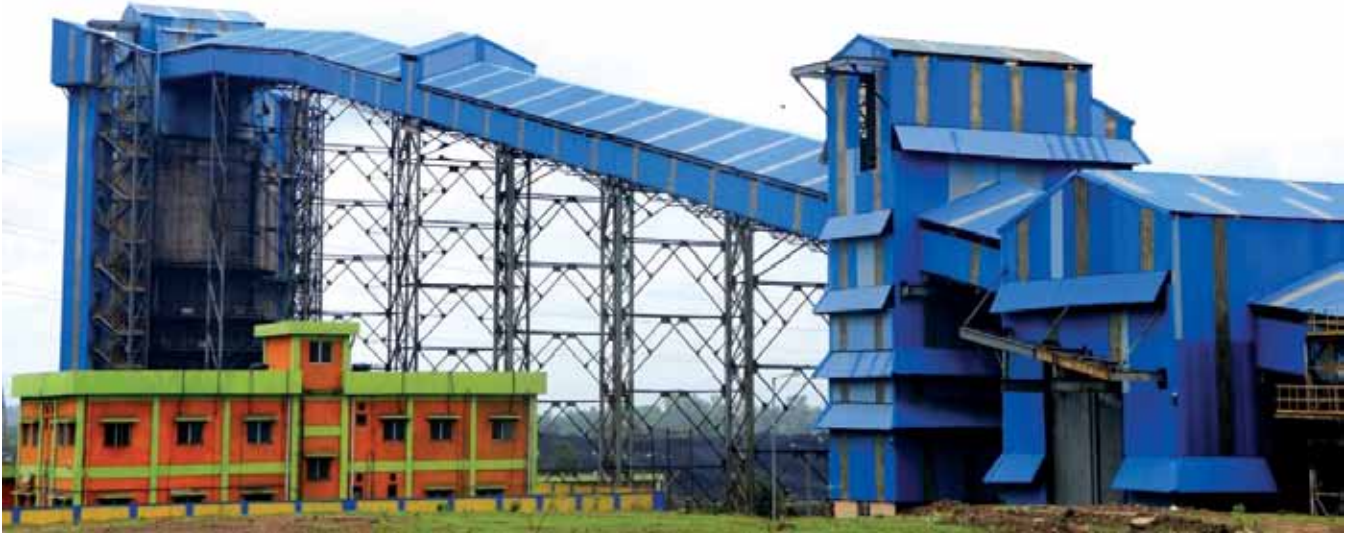
Fig. Silo in Lingaraj OCP in MCL
