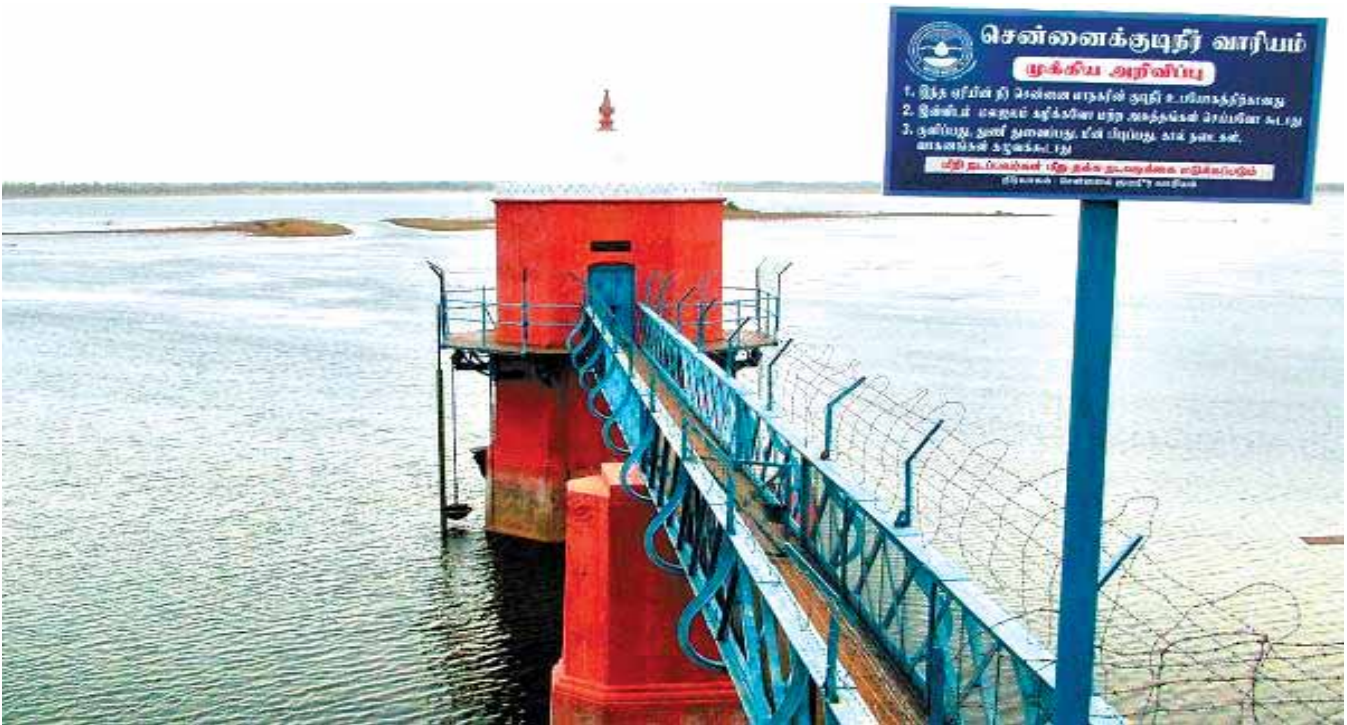
Fig. Water treatment Plant - NLCIL
