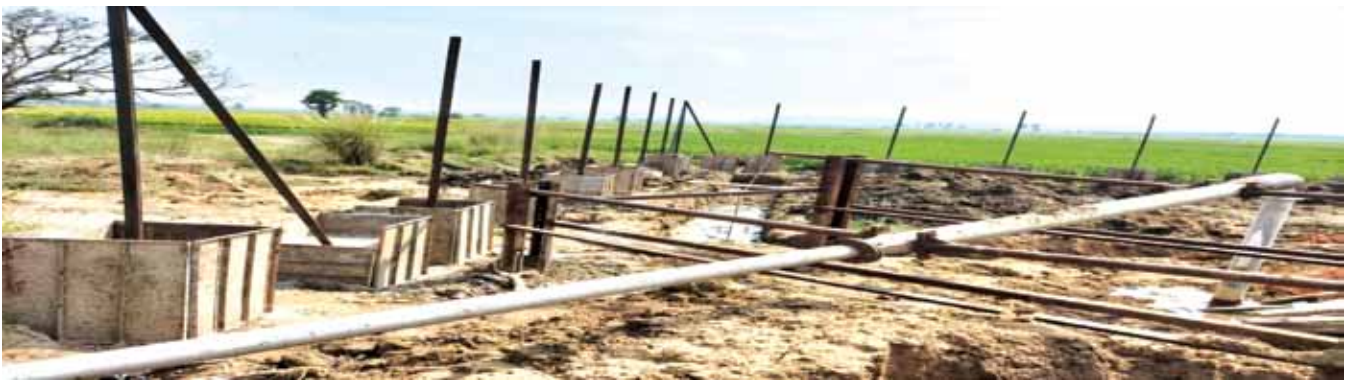
Fig. Work under progress for 20 KW Geo-thermal Project - SCCL
