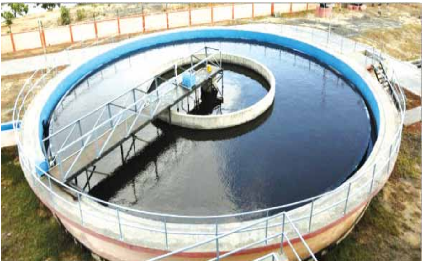
Fig. ETP in Block - B OCP of NCL
