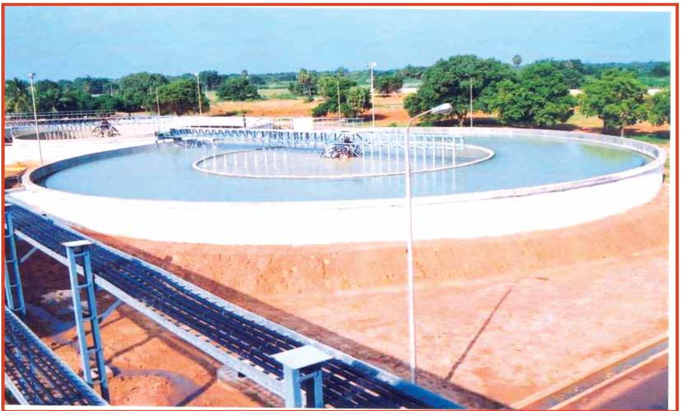
Fig. 180 MLD Treatment Plant at Vadakuthu (Veeranam)
