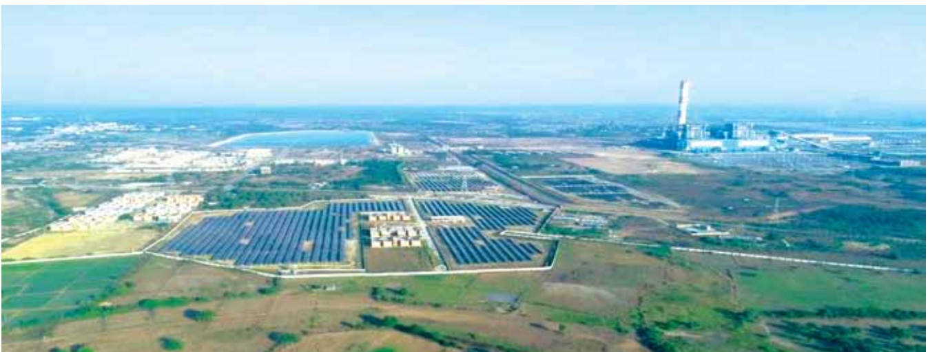
Fig. Sola Power Plant at STTP (10MW)
