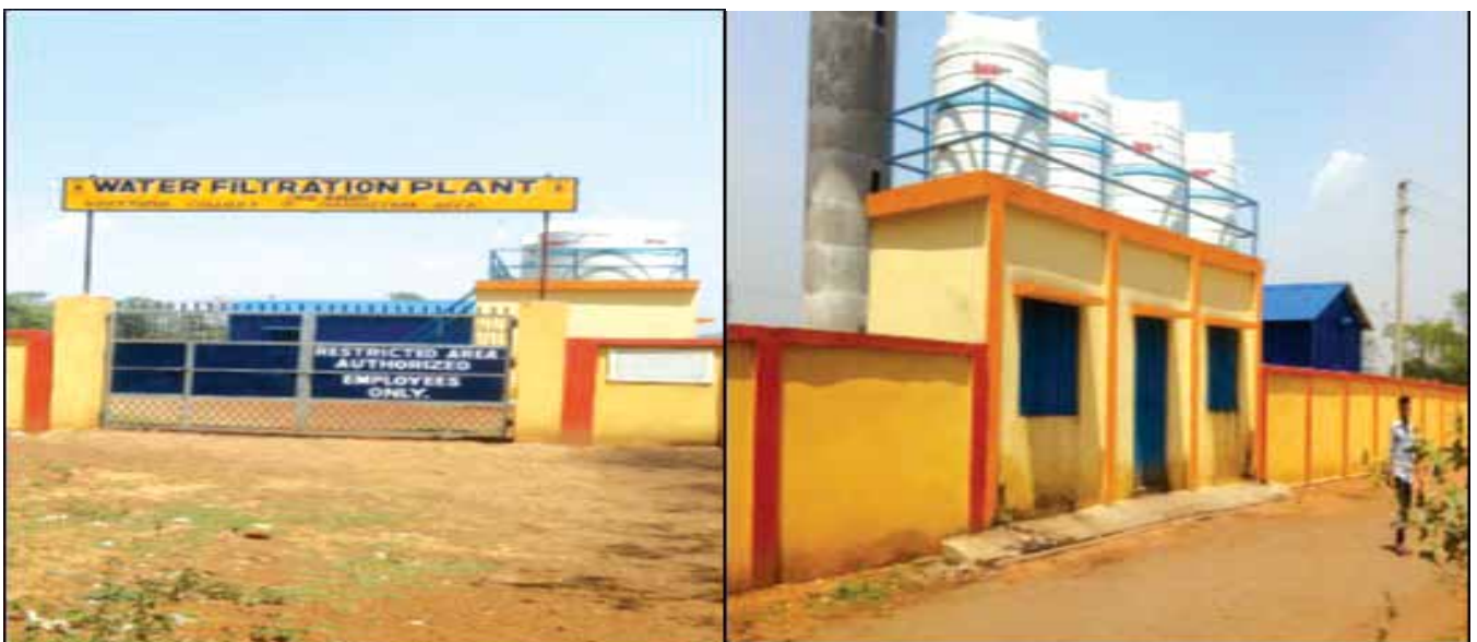
Fig. Water Filtration Plant at Khottadih colliery Pandaveswar Area, ECL
