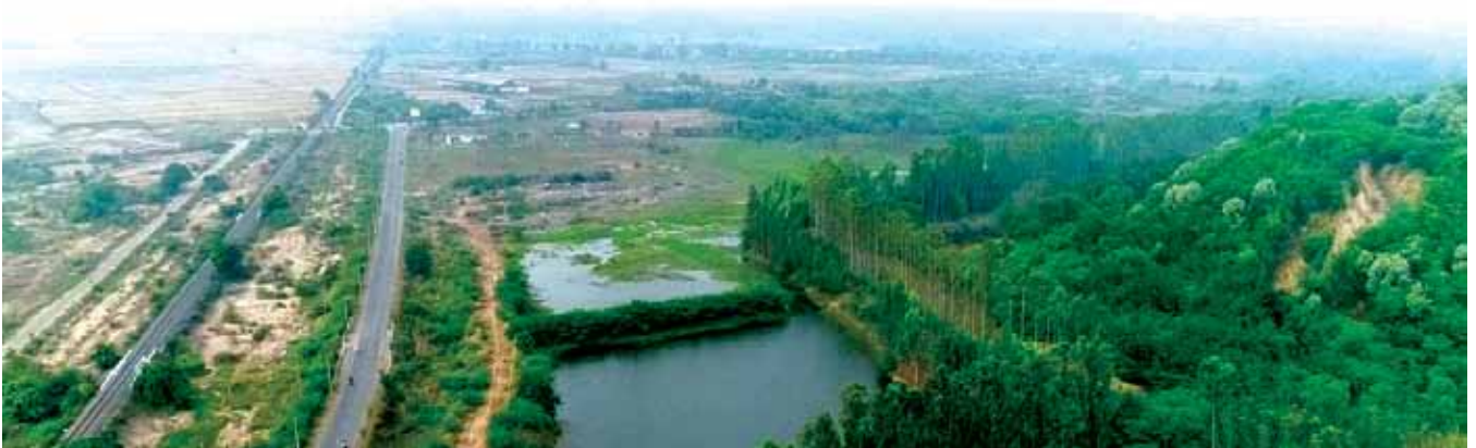
Fig. Summer Storage Tank near RG OC-III project of SCCL
