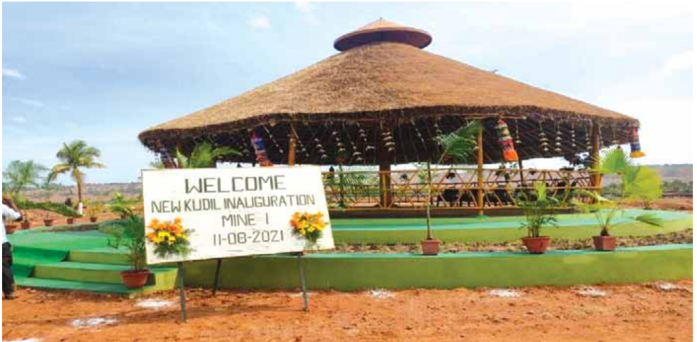
Fig. New Cafeteria in Reclaimed area of Mine-I.
