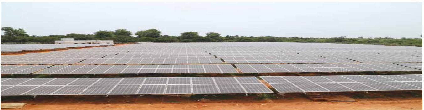
Fig. The flat panel Multi / Poly crystalline silicon PV cell technology in Neyveli Township Block-4
