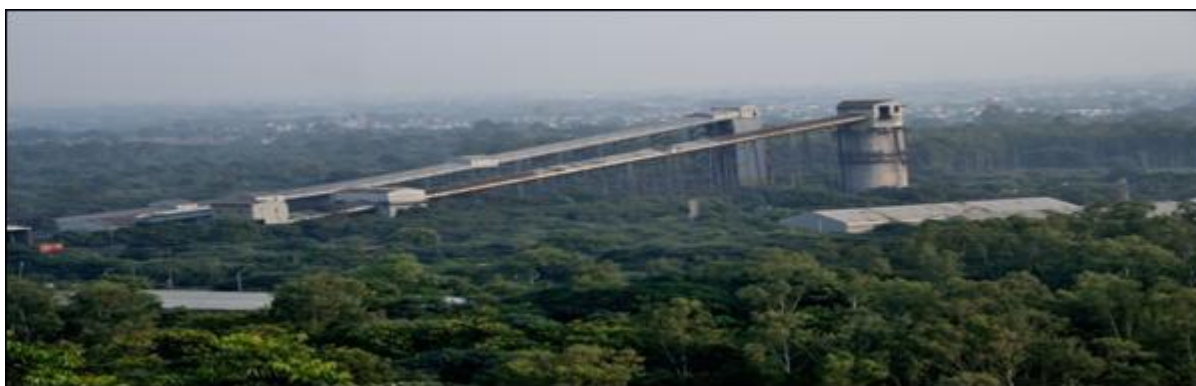
FMC Project at Nigahi OC of NCL – Rapid Loading with closed Belt Conveyor
