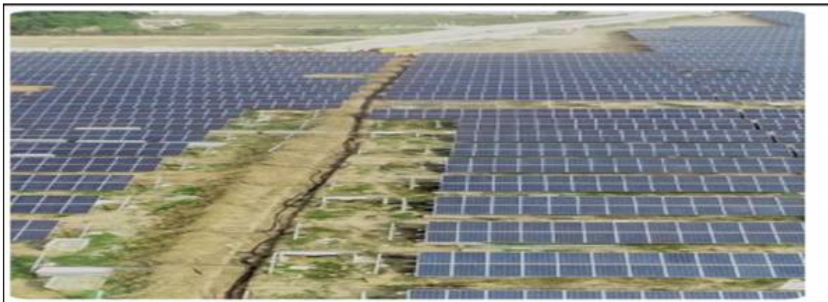
Solar Park (30 MW) at Manuguru, SCCL
