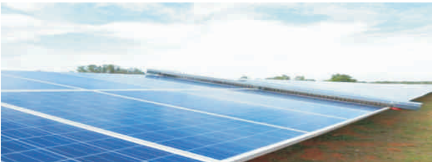
Fig. The flat panel multi/poly crystalline silicon PV cell technology in Neyveli Township Block-4
