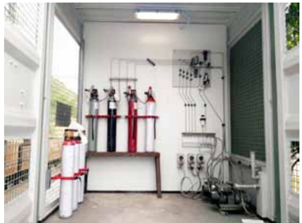
Tube Bundle System in operation at Adriyala Longwall Project
