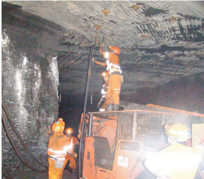
Mechanised Roof Bolting Operations in Underground Coal Mine
