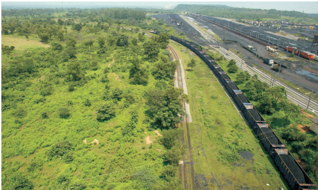
Railway Siding for Coal
