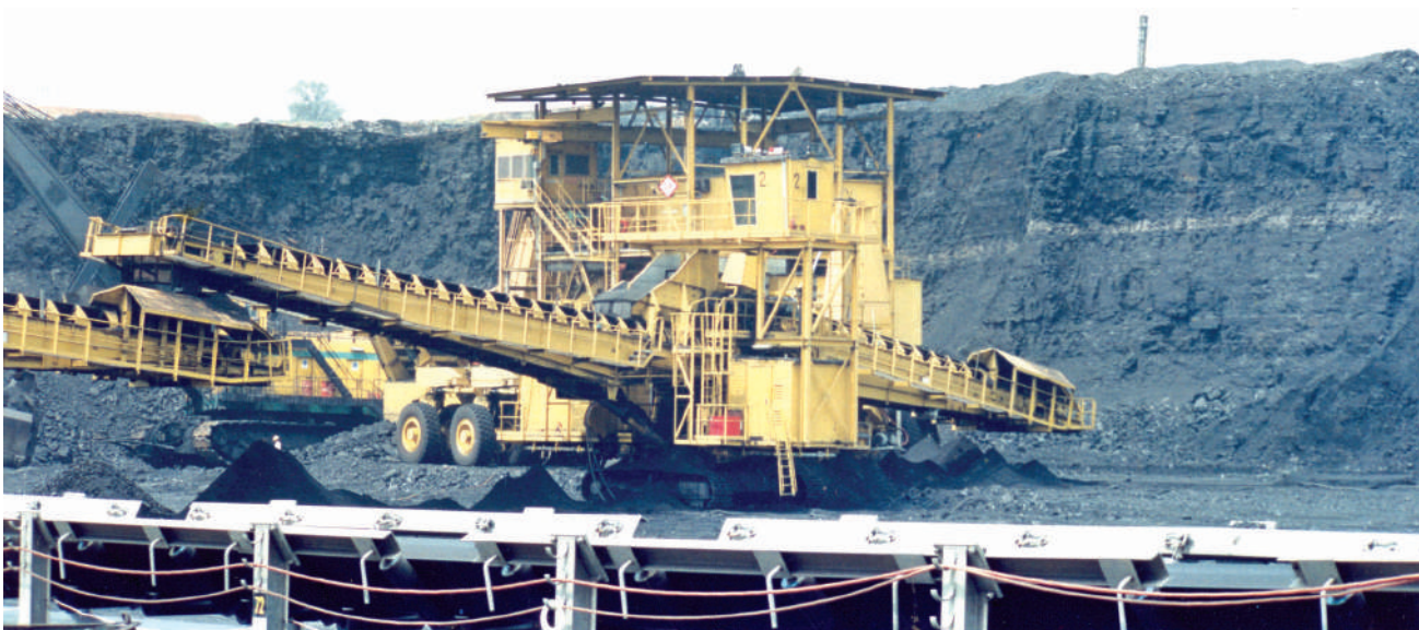
Open-cast mining machine, In-Pit Coal Crusher loading coal on conveyer belt, in open-cast coal mine
